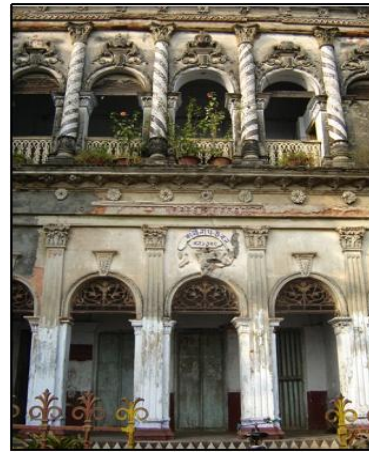
(Source: Field Study, 2006) Figure 26: Previous Front View of Kashinath Bhaban
