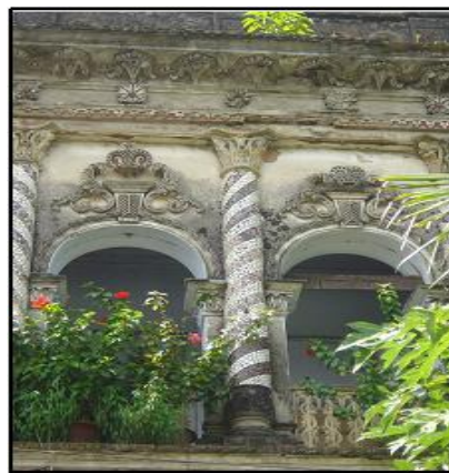
Figure 13: Plaster Decoration and Chinitikri Work of the Front Façade
