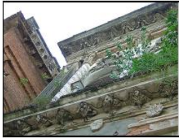
(Source: Field Study, 2006) Figure 5: Projected Cornice Expressed Floor Levels
