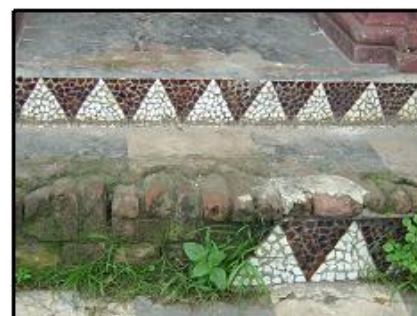
Figure 14: Use of Decorative Colored Broken Tiles on the Step Riser
