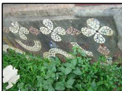
Figure 14: Use of Decorative Colored Broken Tiles on the Step Riser
